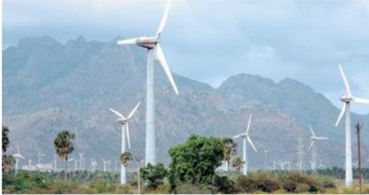
The electrical generators used on wind turbines in sites like Muppandal, produce an output AC of 240 V and a frequency of 50 Hz even when the wind speed is fluctuating. A transformer may be required to increase or decrease the voltage so it is compatible with the end usage, distribution or transmission voltage, depending on the type of interconnection.
